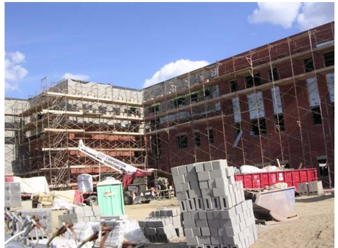
Mason scaffolding around building footprint.
